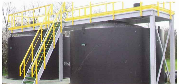
Entrance platforms Water treatment plant
