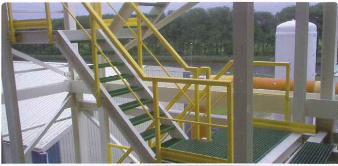
Customized secondary structures Fertilizer plant
